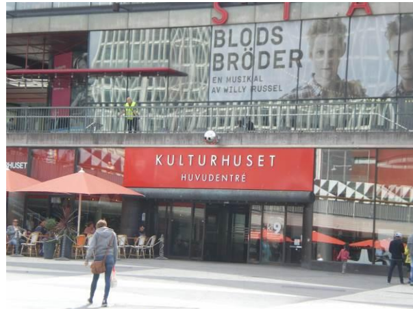
Figure 15: View on the entrance of Kulturhuset from Sergels Torj.
